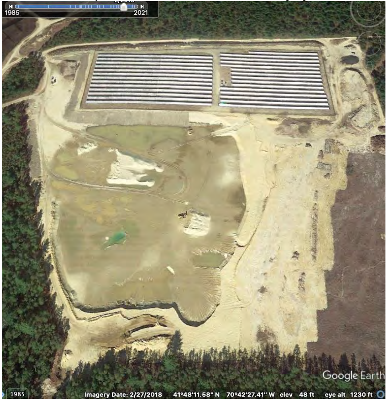
Below: February 27, 2018: Phase 1 solar, earth removal, mining in groundwater
