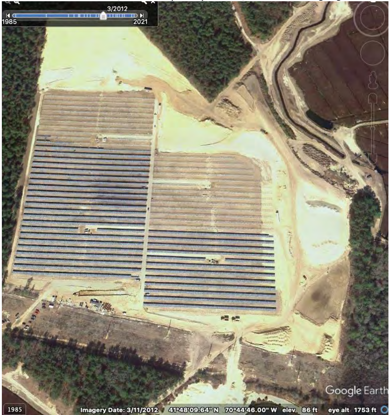
Below: March 11, 2012: Solar partially installed, earth removal ongoing
