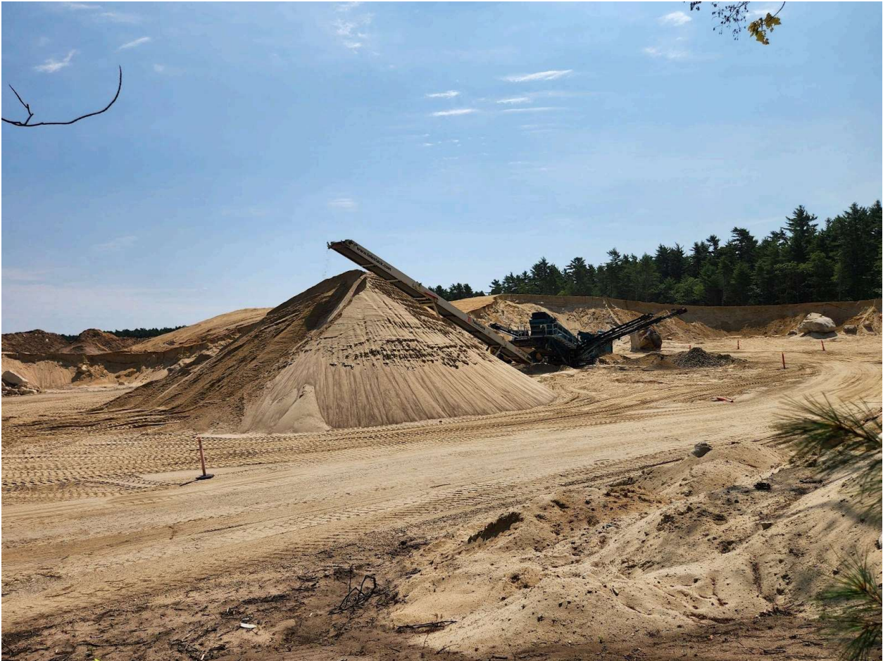
Photo 4: Sand and gravel processing equipment
