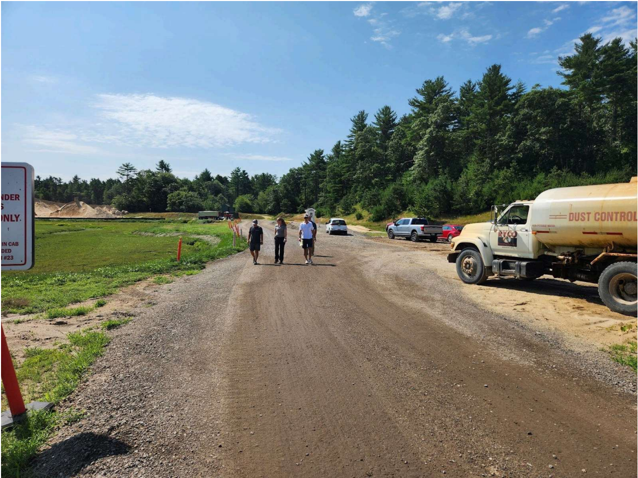
Photo 3: Dust control water sprayer truck
