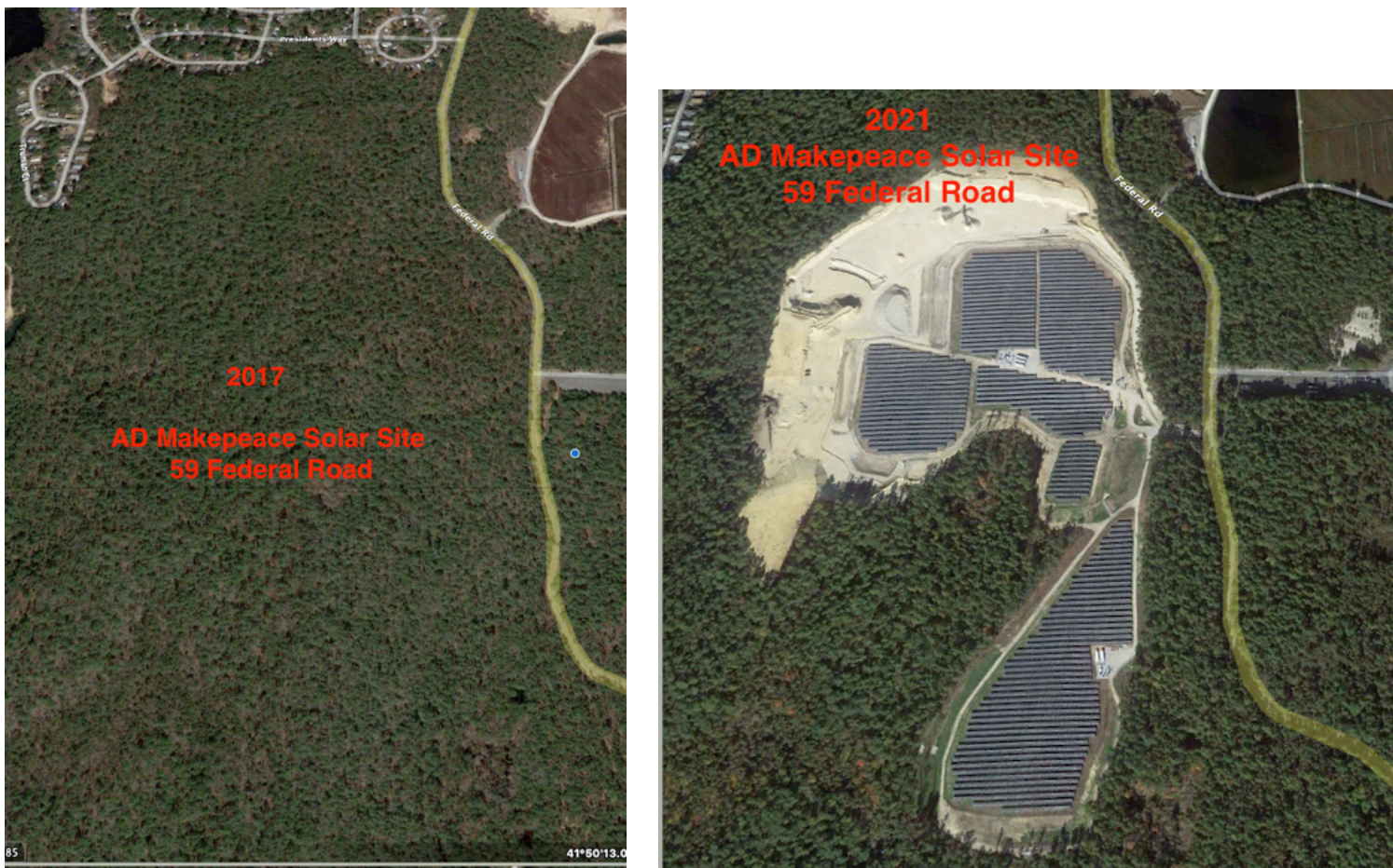
AD Makepeace Solar Site on 59 Federal Road in Carver, MA before and after solar installation
